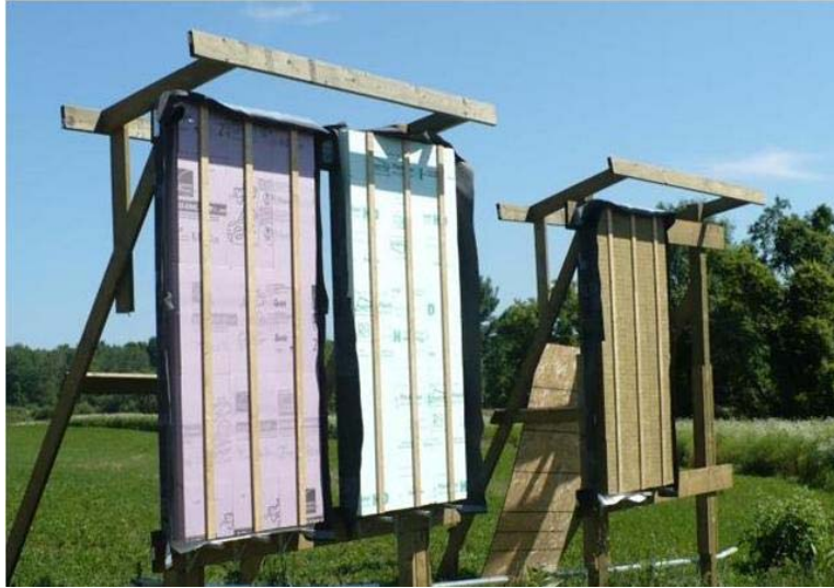
Figure 20. Test wall assemblies under construction
