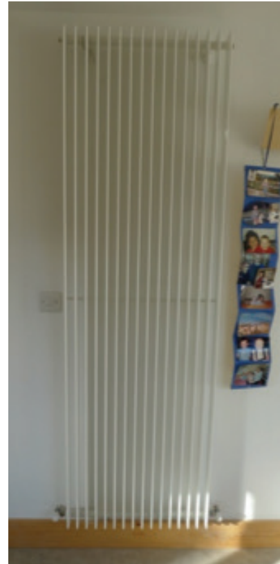
Radiators can be an excellent match for Passivhaus if sized correctly. Photo: Alan Clarke
