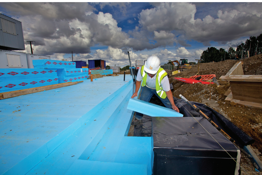
ABOVE: Insulation being installed below the floor slab Photo: DOW Building Solutions
