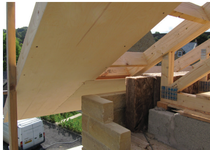
Detail under construction on-site. Photo: Green Building Store
