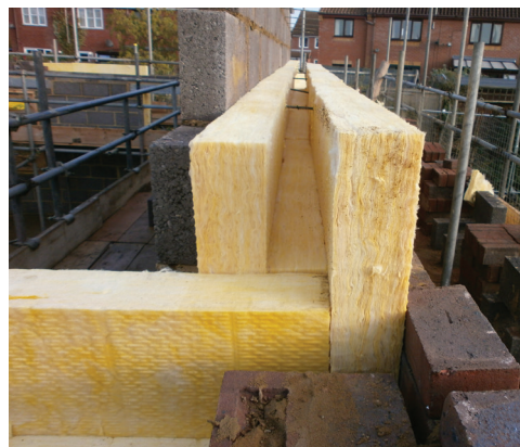
ABOVE: 300mm full-fill cavity with soft fibrous insulation. Photo: Parsons + Whittley Architects
