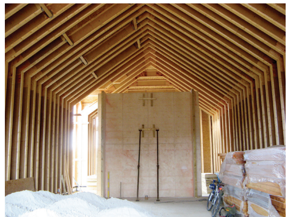
BELOW: I beam portal frame Photo: Conker Conservation
