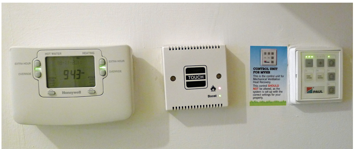
Wall stickers at Gento's Passivhaus Racecourse Estate. Photo: Alan Clarke
