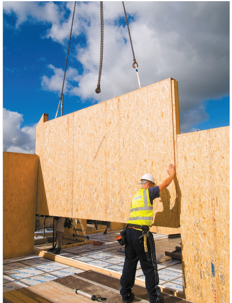
SIPs wall being craned into place Photo: Kingspan Insulation
