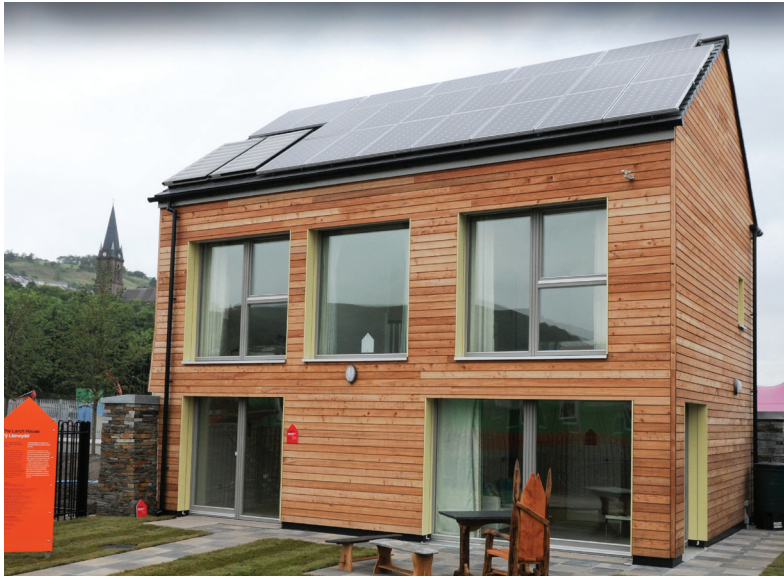
Larch House, Ebbw Vale, using both PV and Solar thermal Photo: bere:architects
