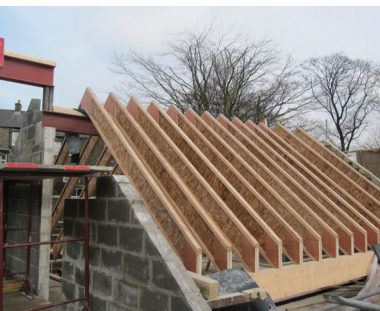
External view of a 'Cathedral' style roof under construction
