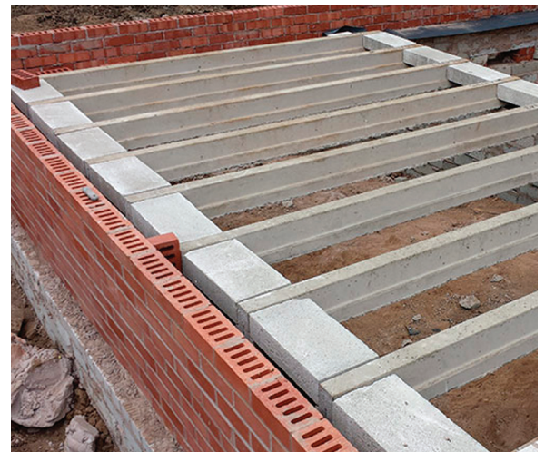
ABOVE: Beam and block floor construction Photo: Total Concrete Products Ltd
