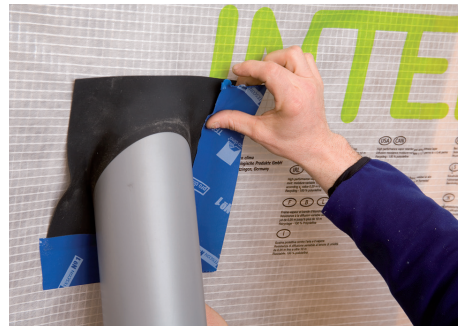
LEFT AND RIGHT: Sealing pipes and cables. Images: Ecological Building Systems
