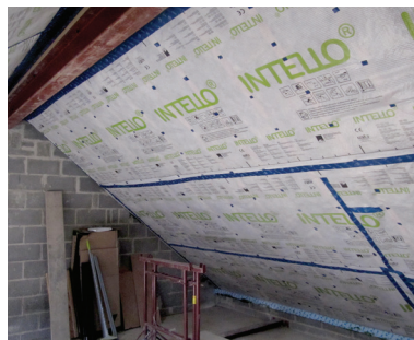
Internal view of a 'Cathedral' style roof under construction Photos: Green Building Store
