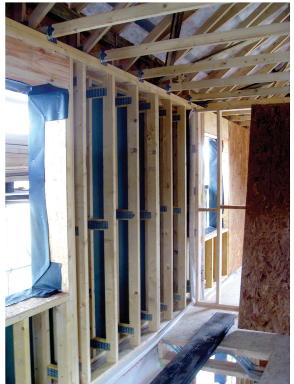
ABOVE: Larsen timber trusses Photo: Eco Arc Architects
