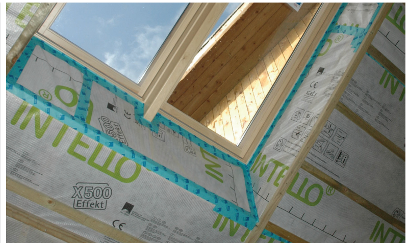
ABOVE: Airtight membrane fixed internally. Photo: PYC Insulation
