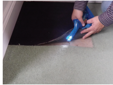
Using chemical smoke to check for leakage between upper floorboards
