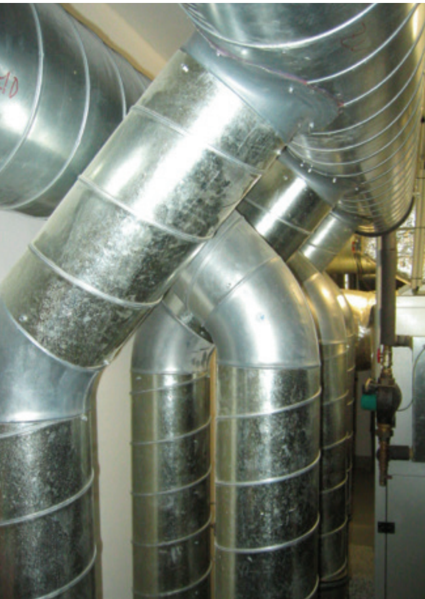
Spiral wound galvanized steel – Efficient, robust, cleanable Photo: Alan Clarke
